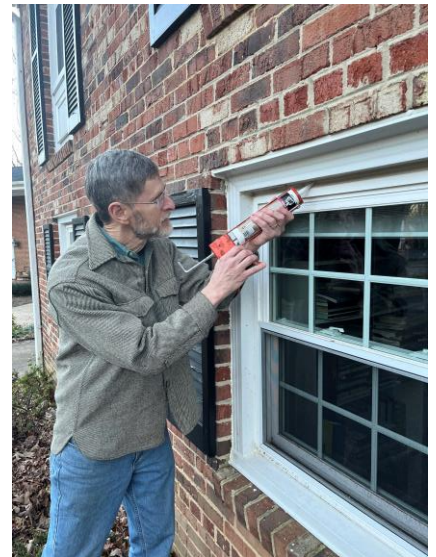
Tom fixing leaks around his window.
