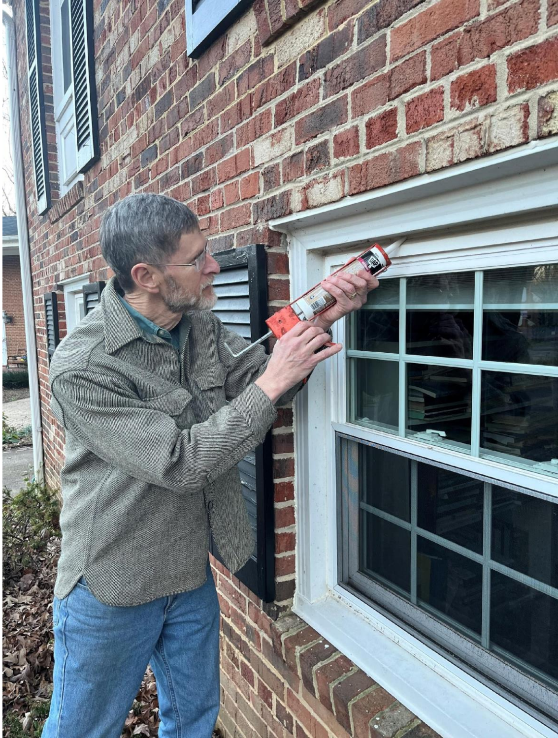
Tom sealing windows to prevent loss of conditioned air.
